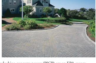
water runoff to control non-point source pollution. Permeable interlocking concrete pavers (PICP) are an EPA-recommended infiltration BMP that filters runoff through aggregate and soils to reduce pollutants.
