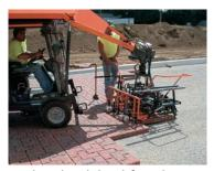
The Eco-Stone® Family of Permeable Pavers features shapes that offer the highest degree of interlock and have been tested and proven worldwide. They are designed for fast mechanical installation, saving time and money on construction, and when
